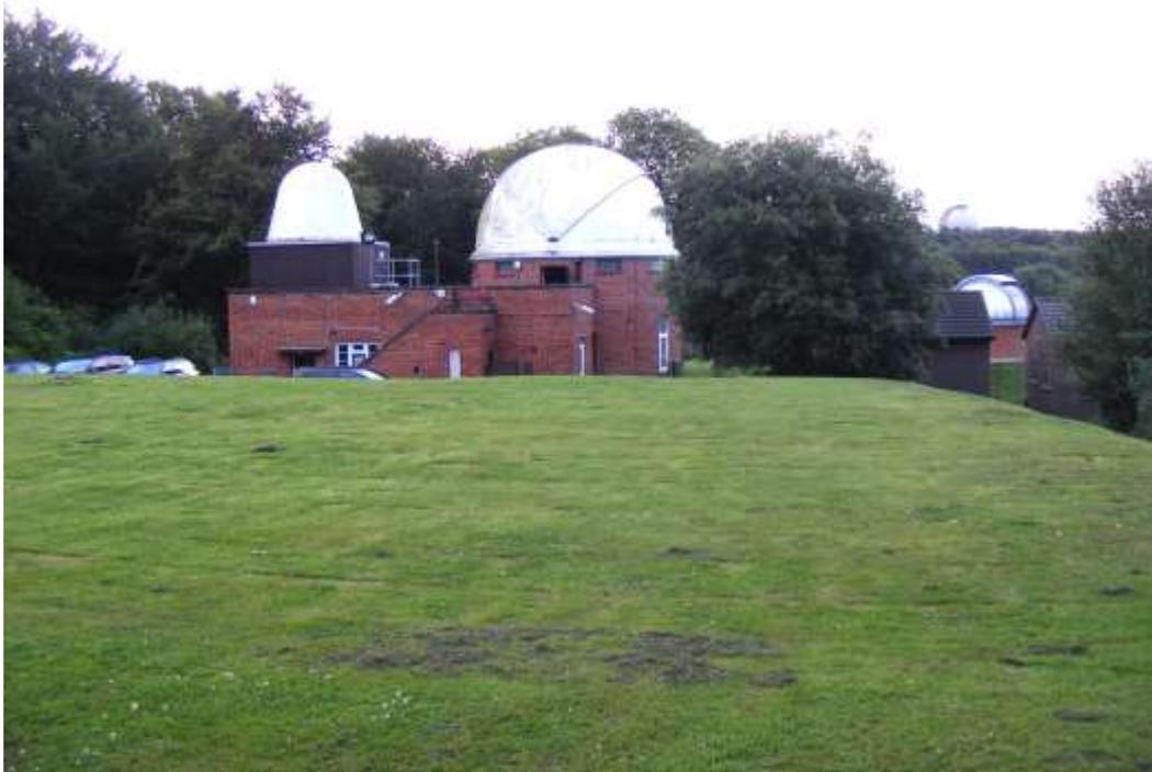
The Space Geodesy Facility at Herstmonceux with the old Isaac Newton Dome in the distance. The main dome of the Facility houses the laser ranging equipment. The smaller dome to the left is an aircraft warning radar that shuts the laser off if an aircraft is detected
